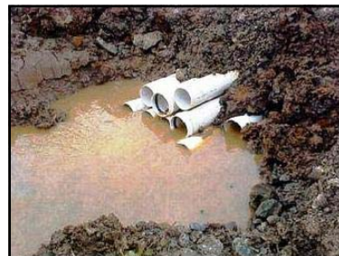
Foto 3: Piping at Marina Bypass
