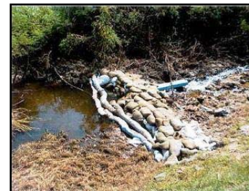
Foto 1: Dike at Forrestal/Langley Drive
